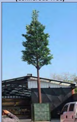
Stealth Installation (Coniferous Tree)
