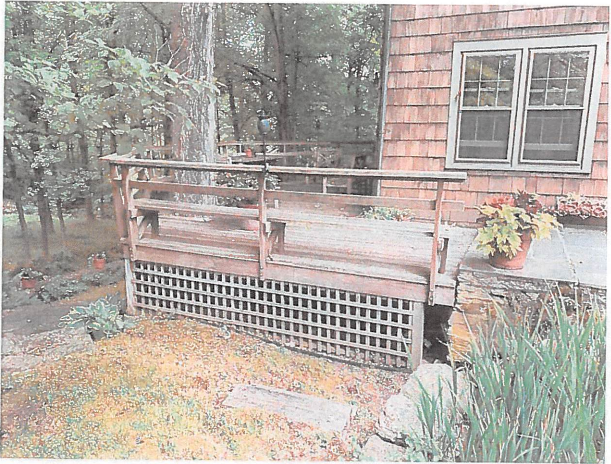
The large tree in the deck will be removed and the Sunroom will attach to the house behind it.
